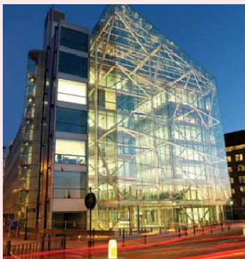
RPC's UK headquarters, Tower Bridge House
